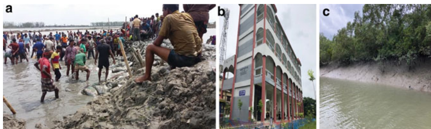
Fig. 5.8 a A recently built embankment after cyclone Amphan through community people for coastal flood protection; b a multipurpose cyclone shelter center; and c coastal mangrove arboriculture
