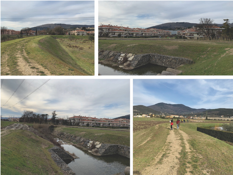
Fig. 1. State of the art of the current area intended for the Carpugnane park.
