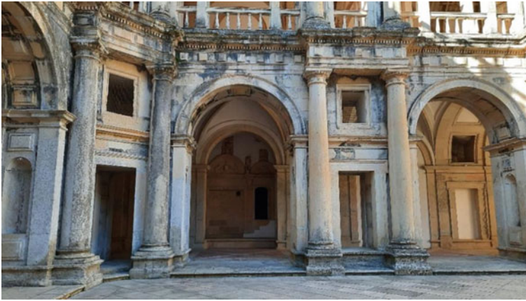
Fig. 10.1 South elevation of the Main Cloister of Convent of Christ in Tomar
