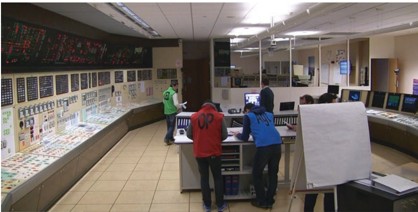
Fig. 15.1 Example of simulation training for the piloting of nuclear reactors (hour-based simulation)—control room in the 900MW reactor
