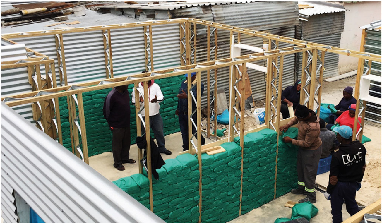
Fig. 5 More than a building site
