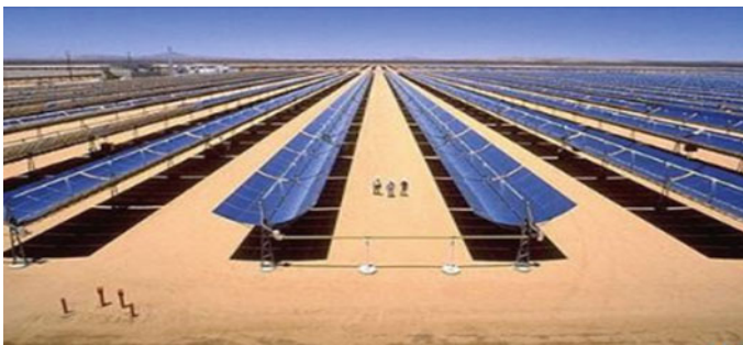
Fig. 2 NOOR 1 (CSP) installation
