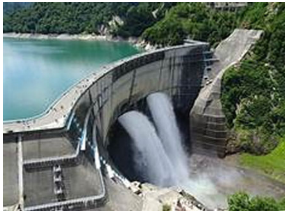
Fig. 2.1 Falling water at Kurobe Dam Spillway, Japan
