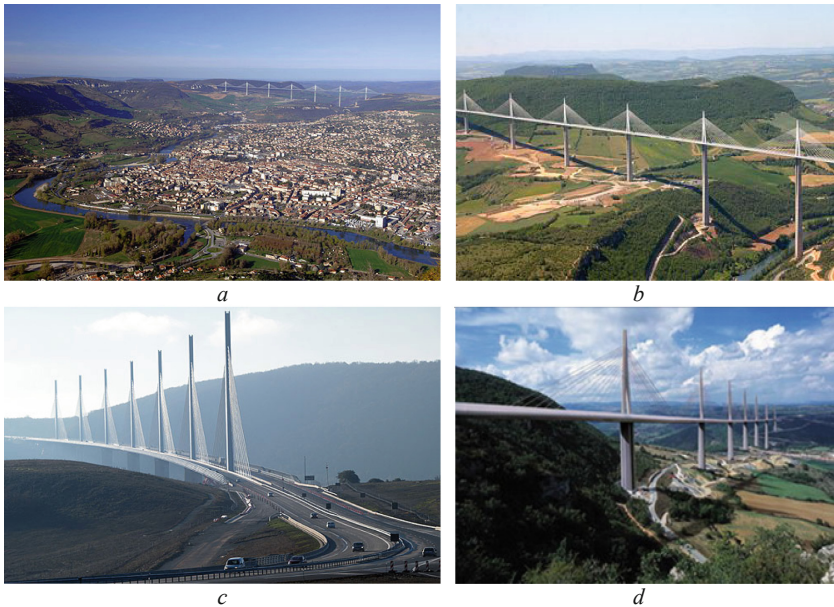
Fig. 2. Panoramic views of the Millau viaduct from the eastern (a), north-eastern (b), south-western (c) and south-eastern (d) sides.
