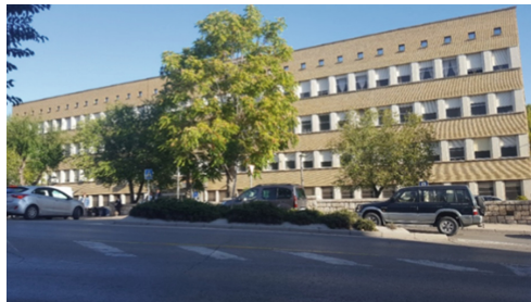
Fig. 3. Overview of the Diagnostic and Treatment Center of the HUIJ.
