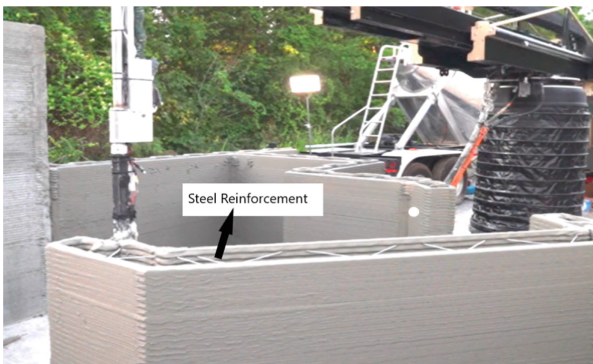
Fig. 2. Application of external reinforcement arrangements [23]
