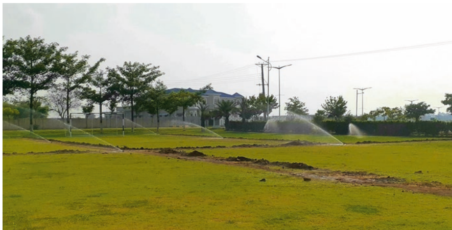
Fig. 4 Sprinkler irrigation system
