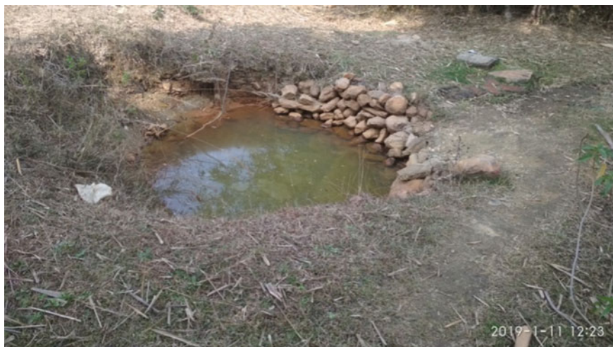
Fig. 16.12 Doba structure at Bela village of Bela GP in Balarampur block
