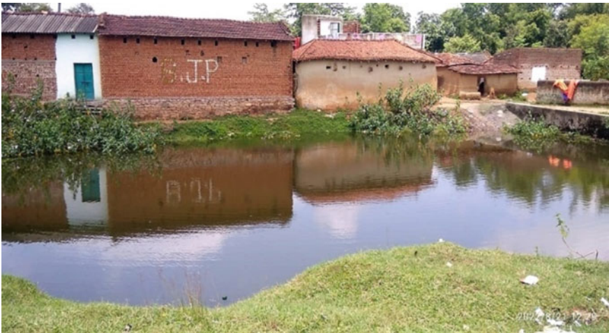
Fig. 16.11 Goira structure in village Chakra of Lagda GP in Purulia-I block
