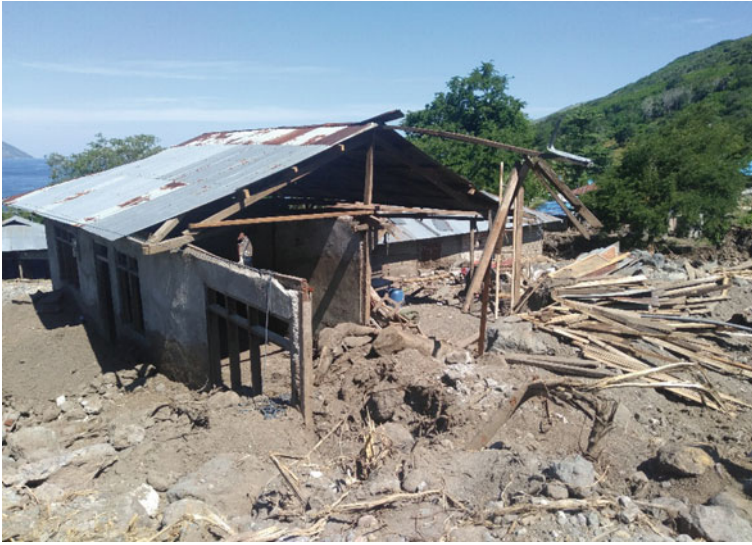
Fig. 21.3 Condition of the house affected by the disaster
