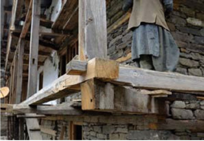
Fig. 24.36 Corner detail: Cantilevered wood supports notch-and-lap-joined wood at the corner. Source Himalayan Vernacular: Kath Kuni, Architecture Visual and Material Arts, 2018
