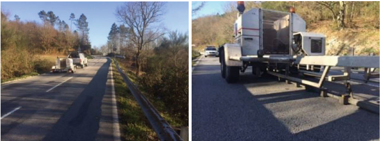
Fig. 3 Aspects of the field trial and FWD testing
