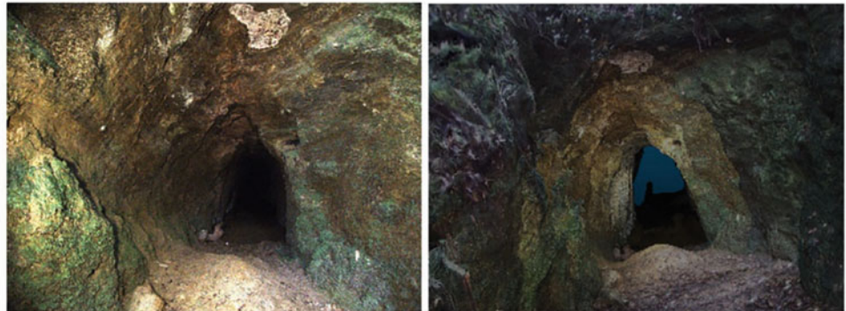
Fig. 6 Aveleiras mine entrance: the image is taken from one of the cameras, and on the right is displayed the corresponding 3D reconstruction
