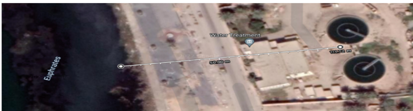
Fig. 2. WTP-1 located at the Riverbank about 111 m
