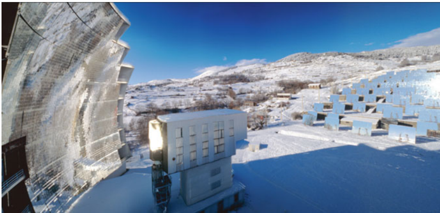
Fig. 8.8 Photograph of a large parabolic mirror in PROMES CNRS, France: the heliostat field reflects their incident direct solar radiation onto a parabolic mirror, which concentrates the solar radiation onto a target at its focal zone
