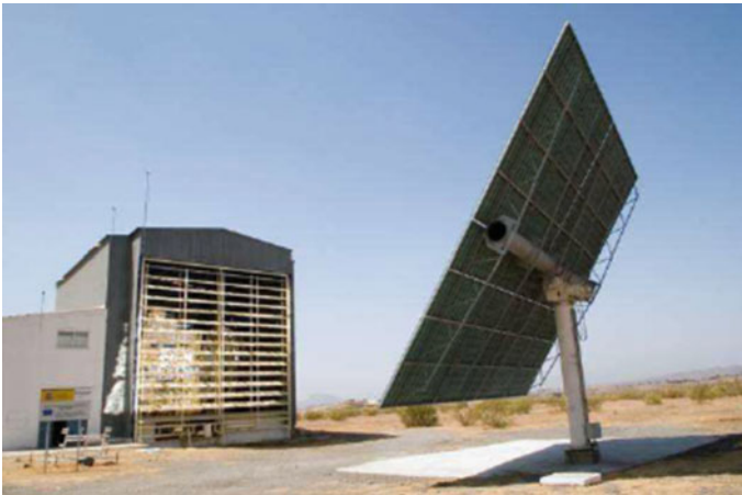
Fig. 8.7 Photograph of a heliostat tracking the Sun and reflecting the solar radiation to a medium size parabolic mirror in Almeria solar plant, Spain
