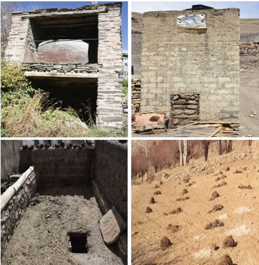
Fig. 10.4 (a) Outside view of traditional toilet in Lahaul and Spiti district. (b) Inner view. (c) Night-soil heaps in agricultural fields
