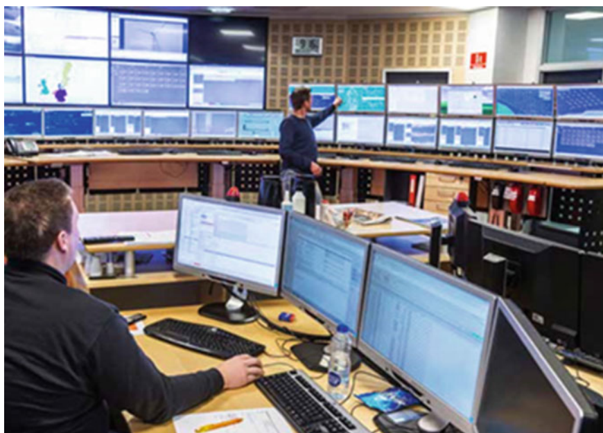
Fig. 16.13 Wind Power Surveillance Centre monitors and operates all turbines. Source Vattenfall Eldistribution
