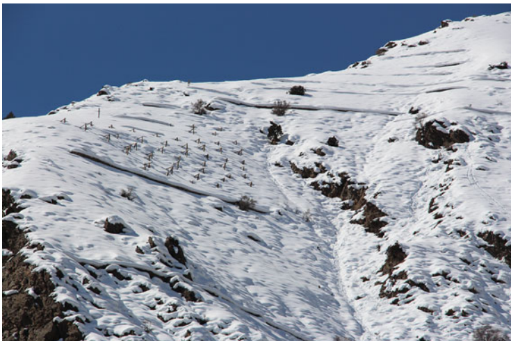
Photo 16.3 Avalanche mitigation interventions (terracing and snow glide tripod) implemented by AKAH Pakistan in Shershal village in district Lower Chitral
