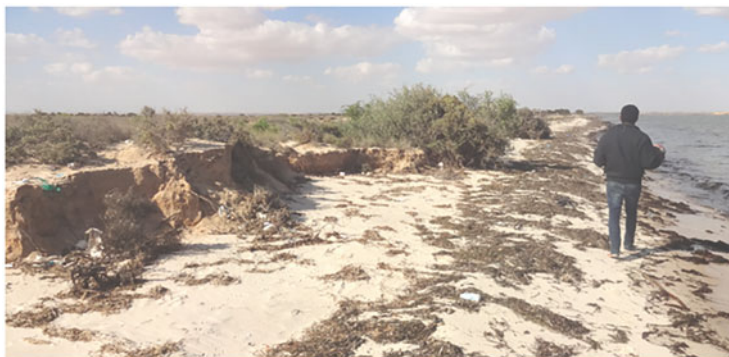
Fig. 12.7 The state of the coast at Bou Said (South Skhira), in an area far from all human intervention. The beach has become very narrow, the foredune is truncated and its vegetation bare (photo Ameer Oueslati, Oct. 2018)
