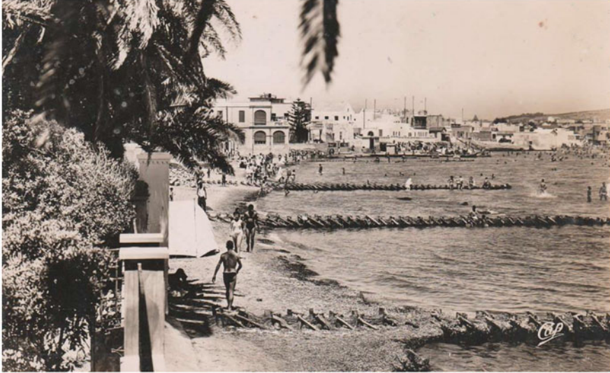
Fig. 12.3 One of many postcards from the first half of the twentieth century showing the narrowing of the beaches in the northern suburbs of Tunis and the wood groins (the original photo is owned by the author)
