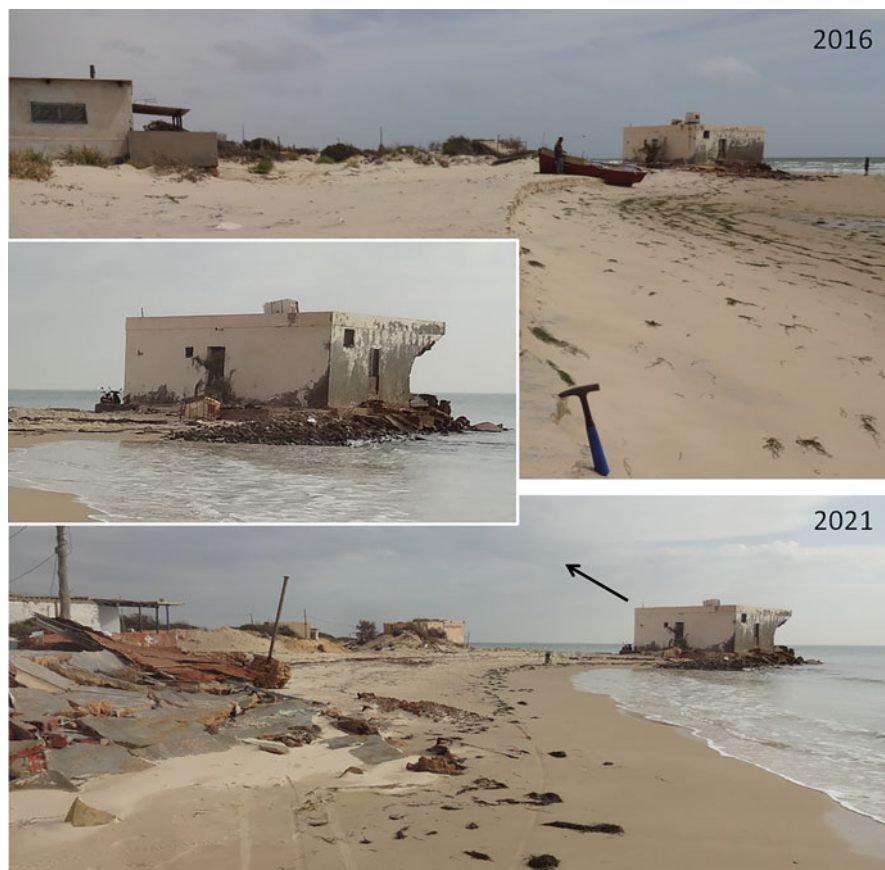
Fig. 12.10 The state of the beach and the recent constructions a few hundred meters from the mouth of Oued Chaffar: the comparison of the photos is revealing as to the significant reduction in the width of the beach and the rate of the shore retreat (Photos, Ameer Oueslati)
