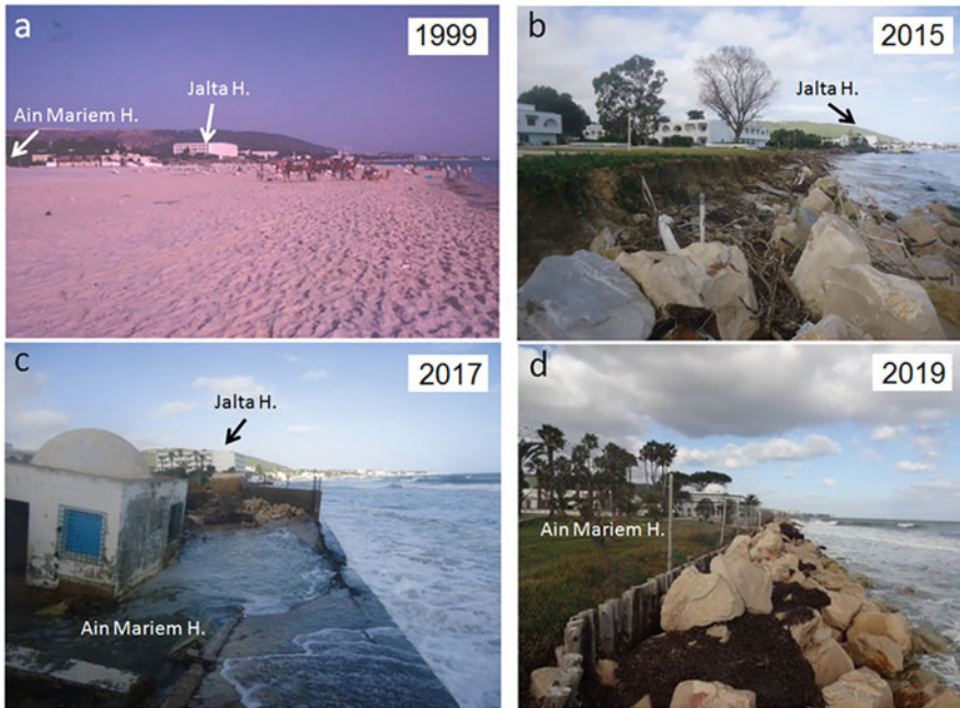
Fig. 12.12 The evolution of the beach between Ain Mariem and Jalta hotels in the space of 20 years (1999–2019) (photos, Ameer Oueslati). (a) The beach in 1999; (b) disappearance of the beach and formation of a small cliff showing allogenic materials on the sand of the beach and the foredune; (c) the situation towards the end of a storm in November 2013; (d) the current situation; the place is given to protective structures
