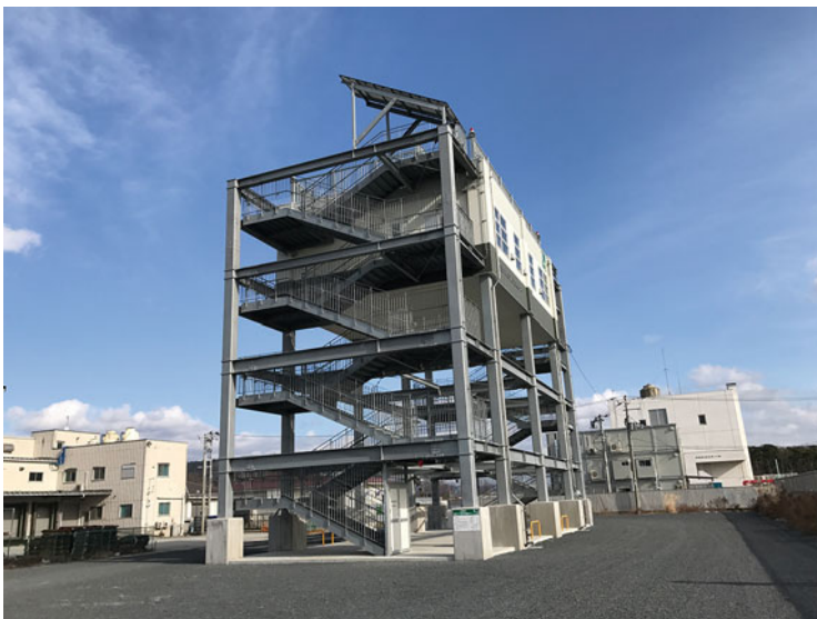
Fig. 15.3 Evacuation tower in Miyagi Prefecture
