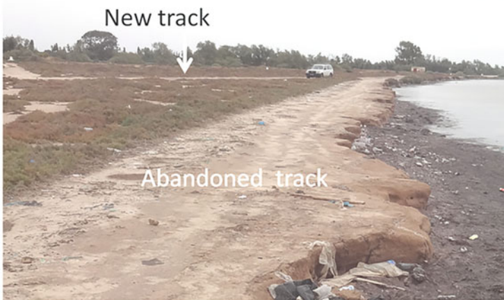
Fig. 12.6 South to Melloulèche (between Mahdia and Sfax): the importance of marine erosion sometimes forced the displacement of coastal tracks. However, the coast is characterized by the weakness of its bathymetry and still away from seafront managements (photo, Ameur Oueslati, Nov., 2017)
