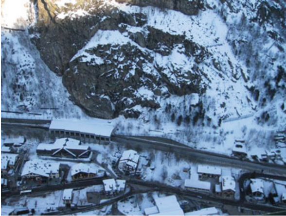
The M. de la Saxe rockfall barriers (west)
