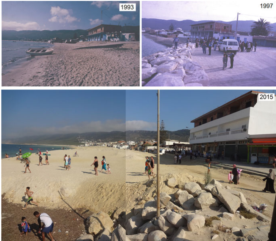
Fig. 12.25 Raf Raf beach, one of the rare beaches to have benefited from important artificial replenishment (the coast of Ejjeimi-Soliman in the Gulf of Tunis offers another significant example). This followed attempts at protection by hard structures. The photos also show the evolution of the situation since 1993. We recognize the same building (unfinished on the first two photos) that serves as a landmark. The rapid erosion is mainly due to the waterfront constructions all built on the foredune (photos, Ameer Oueslati)
