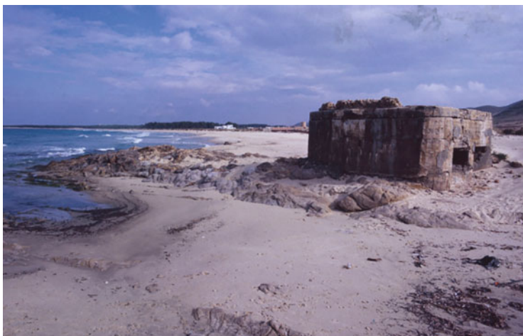
Fig. 12.5 Blockhaus at El El Ghirane, annexed to the foreshore area. It owes its conservation to the fact that it rests on a resistant substratum. Originally, it must have been in the dune area. (photo Ameer Oueslati, July 2015)
