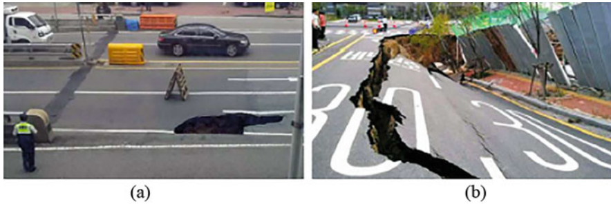
Fig. 1.5 Photographs of urban road sinkholes that were due to an underground void in the area: (a) Seokchon Station in Seoul, Korea (August 2014), and (b) Incheon, Korea (July 2014) (modified from Nam et al. 2018)
