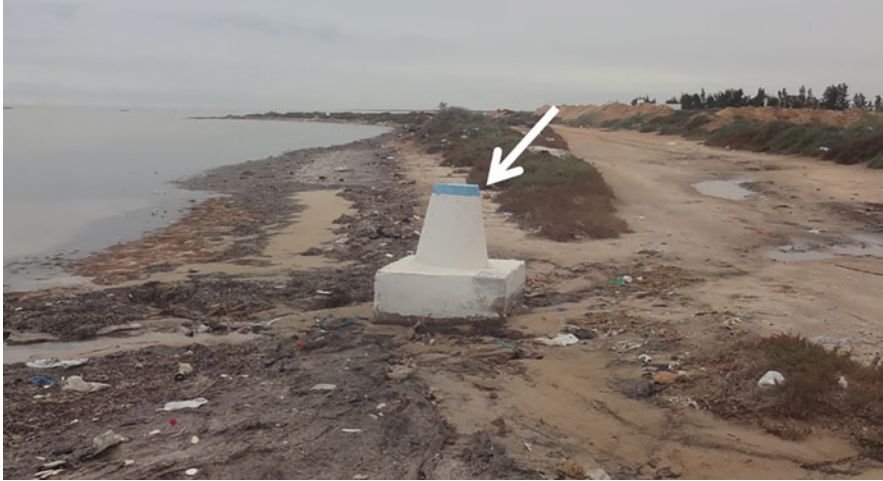
Fig. 12.19 A very recent boundary marker of the Public Maritime Domain located in the intertidal zone (photo, Ameer Oueslati, Nov., 2017). It is already beginning to be dislodged by waves and is overtaken by seawater during storms, as the puddles visible on the track suggest. According to the DPM definition, it must be further inland!
