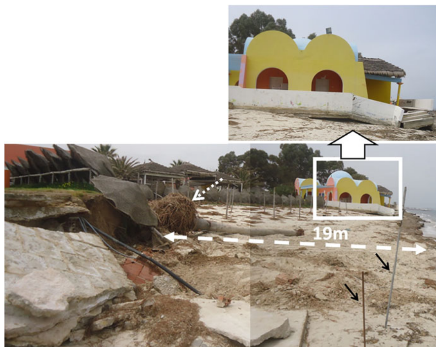
Fig. 12.16 One of the illustrations of the state of the beaches of Skanès coast in the aftermath of the storm in March 2012. 19 m is the width of the space that was part of the hotel enclosure before the storm. It corresponds to the distance which separated the felled palm tree (small dashed white arrow) from the sea. We also recognize the debris and the external limit (dark arrows) of a pool which was originally implanted at the expense of the inner part of the beach (photos, Ameur Oueslati, March 2012)
