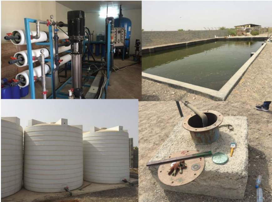
Fig. 2 A desalination system in one of the Omani farms (Al-Batinah region) including the RO system and the evaporation pond to treat the brine
