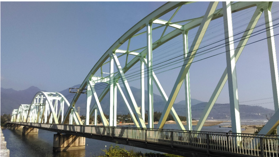
Fig. 2. Nam O railway bridge
