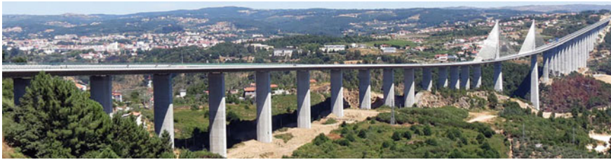
Fig. 10.2 General view of the Corgo Bridge
