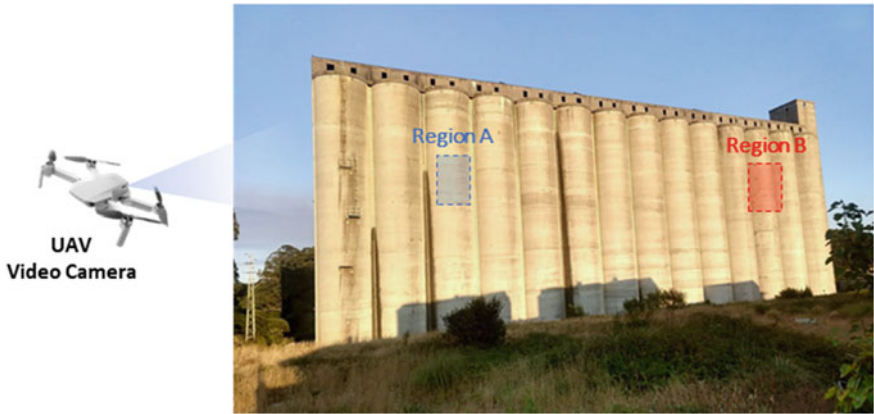
Fig. 6.10 Silo overview with the identification of the inspection regions (A and B)
