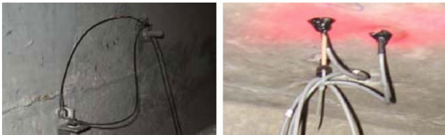
Fig. 12.12 Accelerometers (left) and temperature sensors placed inside the bridge’s cross section
