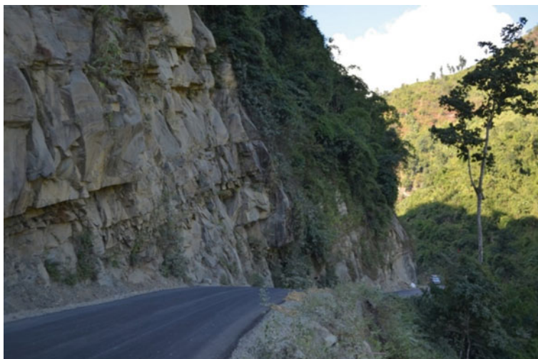
Fig. 7.1 Slope section of Nungkao Landslide showing variable block size due to uncontrolled blasting
