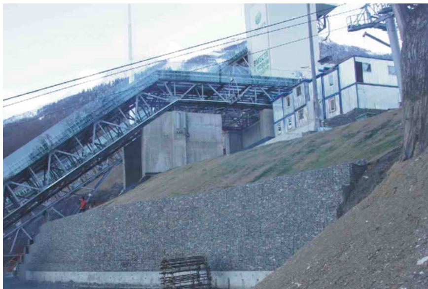
Fig. 12.10 Gabion retaining wall at site “Russkie Gorki”
