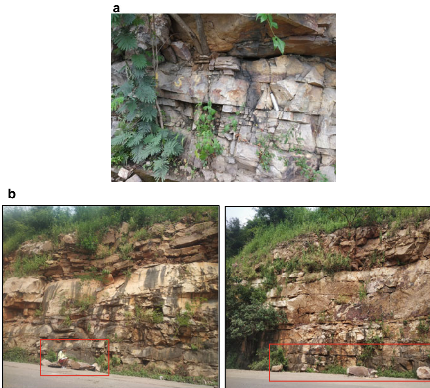
Fig. 4.2 a Rock mass condition at location 1, b Detached blocks lying on the road at locations 2 and 3 (in the red box)
