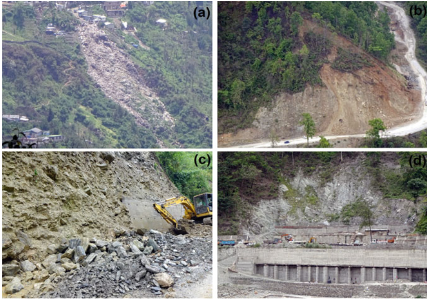
Fig. 16.7 Communication interruption by landslides: a Debris slide in the residential region, b landslide along the national highway, c Rock slide along the transportation network, d Road blockage by landslide in construction site (Field observation 2016)
