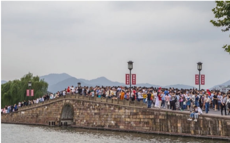
Fig. 2 The broken bridge at West Lake heritage site in Hangzhou
