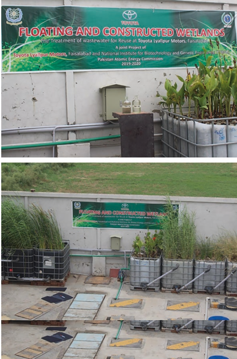
Fig. 4.7 Integration of floating treatment wetlands and constructed wetlands at a car-wash station for the treatment and reuse of the wastewater
