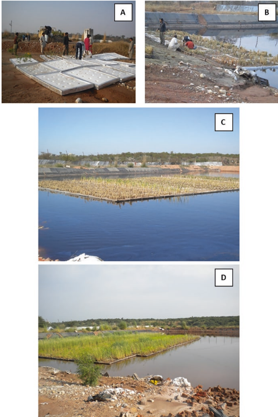
Fig. 4.5 The use of floating treatment wetlands in a wastewater pit for the remediation of crude oil-polluted wastewater of Rajjan Oil Field, Chakwal City, Pakistan. Vegetation of the plant in the mat (a), transfer of the vegetated mats in the pit (b), the growth of the plant at the start (c), and growth of the plants after 6 months of vegetation (d)
