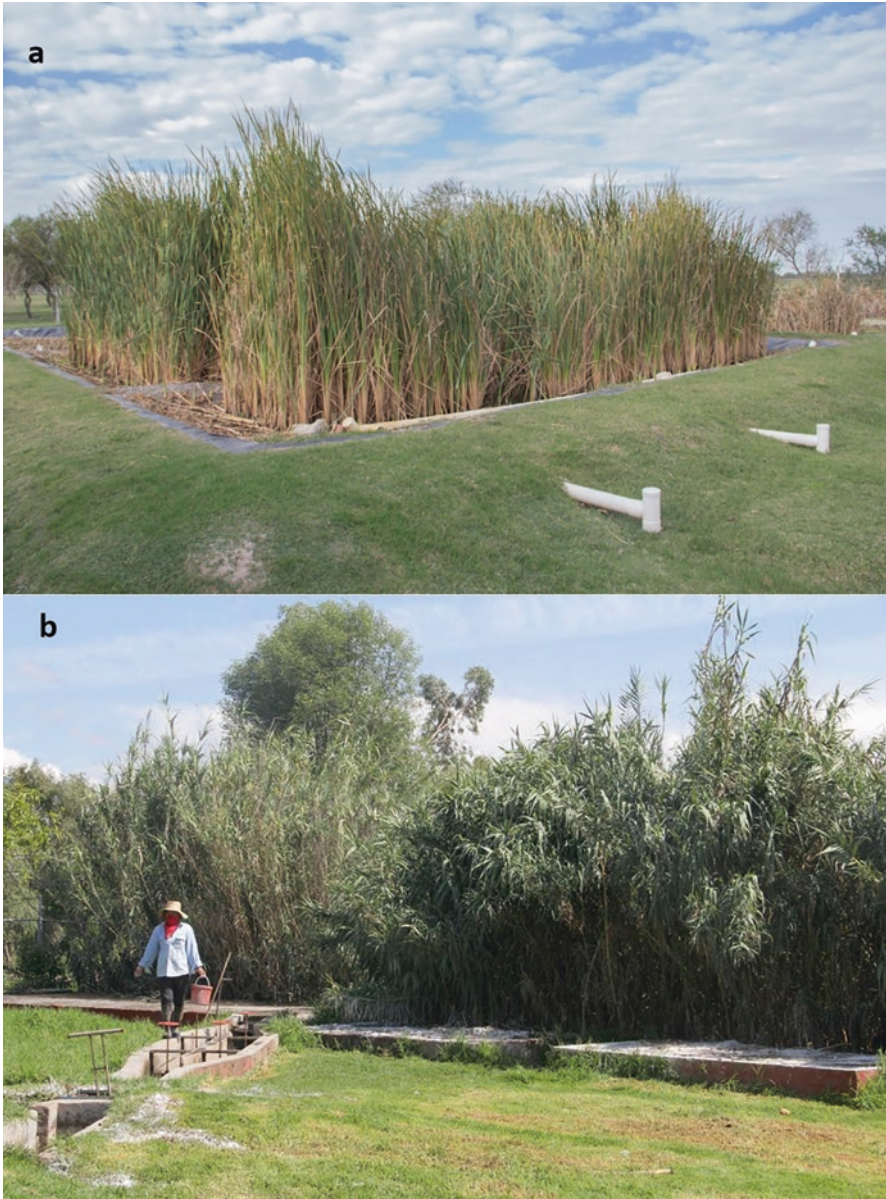
Fig. 3.3 Emergent species used in TWs. (a) Typha domingensis in a constructed wetland for the treatment of effluent from a pet-care center depending on a pet-food factory in Argentina and (b) Arundo donax in a wetland constructed for the treatment of sewage in Mexico (Photos by H.R. Hadad)
