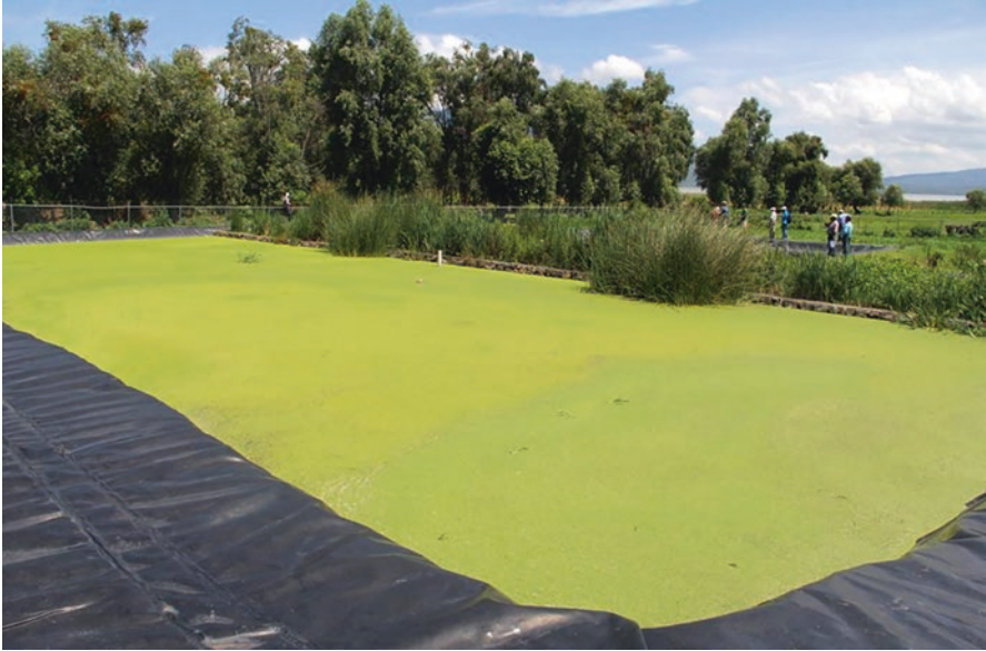
Fig. 3.5 Duckweed invasion in a wetland constructed for the treatment of sewage in Mexico (Photo by H.R. Hadad)
