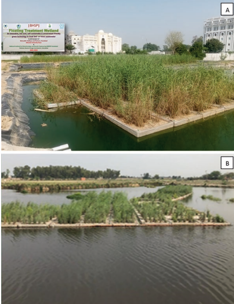
Fig. 4.4 Use of floating treatment wetlands at Akhuwat University, Kasur City, Pakistan (a) and Town of Manak, Lahore City, Pakistan (b), for the remediation of sewage wastewater
