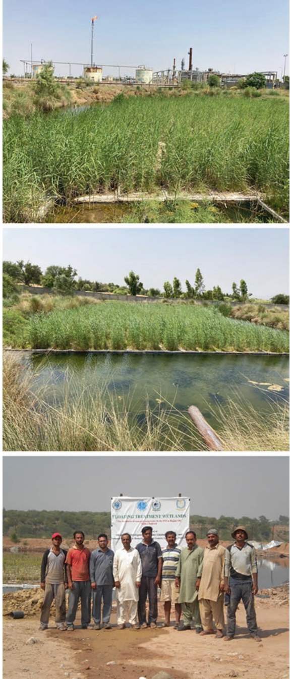
Fig. 4.6 Application of floating treatment wetlands in a pit at Dakhni Gas Plant, Attock City, Pakistan, for the remediation of crude oil-polluted wastewater
