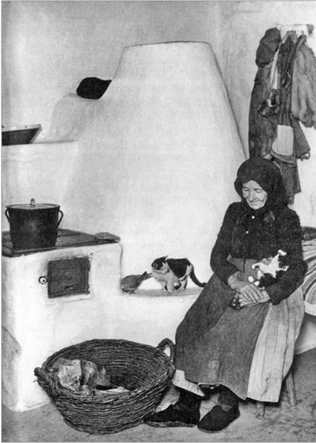
Fig. 15.2 Traditional masonry ovens in Vojvodina (“paorska peć”), retrieved from https://www.ravnoplov.rs/paorska-pec/
