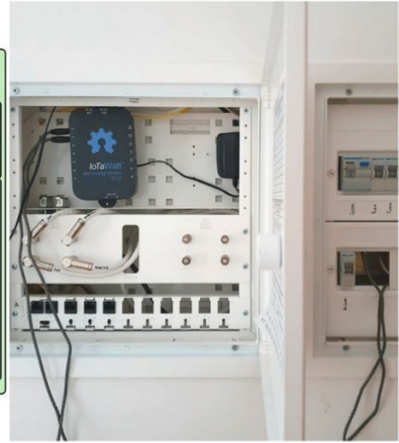
Fig. 2. IotaWatt’s communication interface in the test phase.
