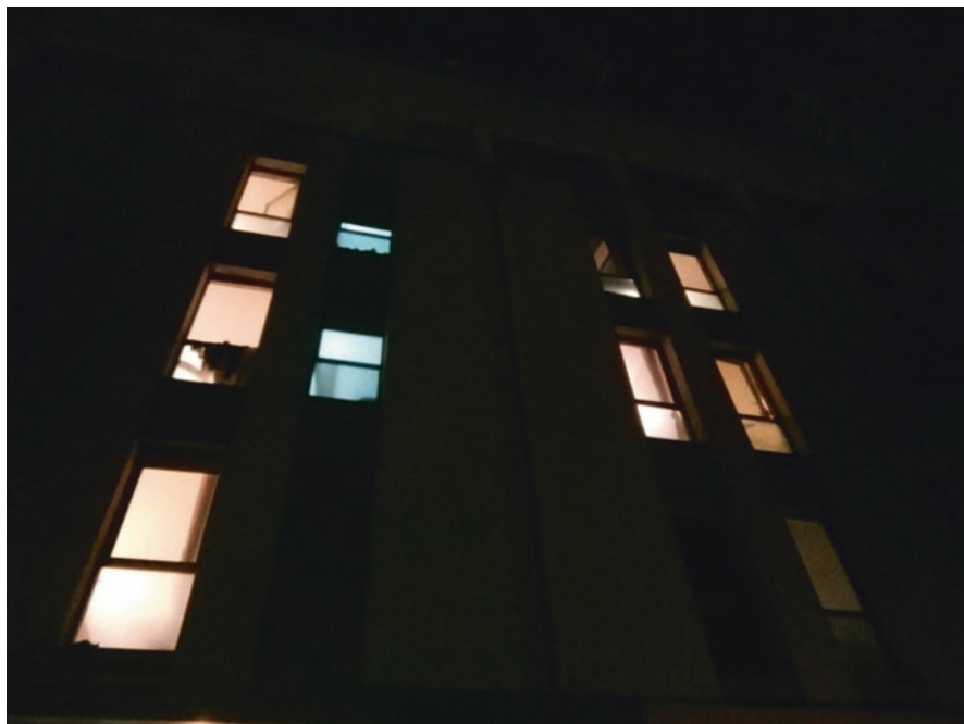
Fig. 7.1 The centre, seen from the outside. (Author's picture)
