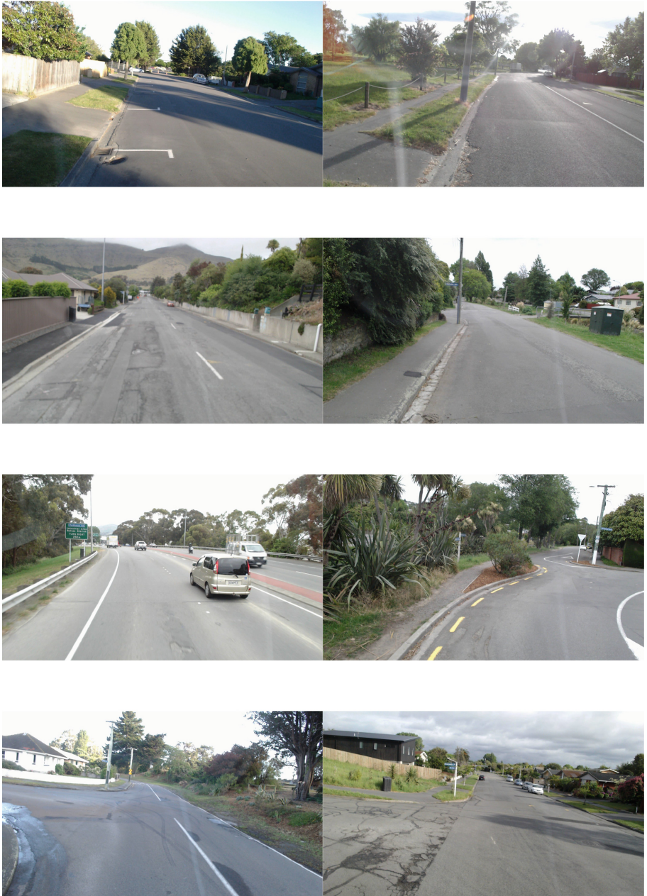
Fig. 6. Detected defect examples, with pothole detection examples in the first two rows and other defects detection examples in the last two rows.
