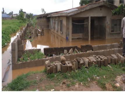
Fig. 9. House submerged by flood. Source: Field survey (2019)
