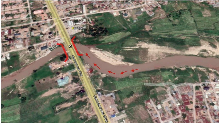
Fig. 1. Change of water course near the bridge (red arrows)
