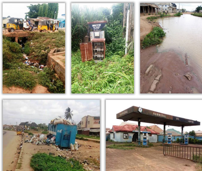
Fig. 8 Examples of resource wastage, poor infrastructure, and high-country risk from real sector development in Ota, Ogun, Nigeria: ( top left ) poor bridge infrastructure, ( top middle ) dilapidated electricity transformer, ( top right ) regularly flooded internal road, ( bottom left ) overflowing waste on urban road, and ( bottom right ) abandoned service station due to poor road conditions. Source: Photographs by Olajumoke I. Omodara, July 31, 2022
