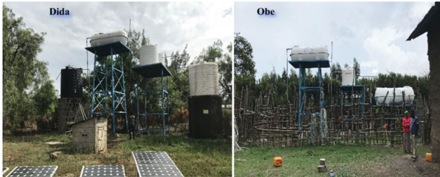
Fig. 4 Treatment plants using zeolite-based technology in two schools of the Salesians Mission (Don Bosco) in the area of Ziway, the central Ethiopian Rift valley
