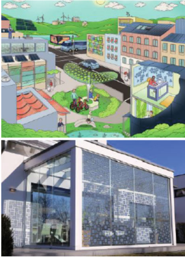
Fig. 3.6 Top: Visionary concept of the OPV product portfolio. Flexible and semitransparent modules are integrated indoors as well as outdoors into windows, facades, installations, greenhouses, urban mobility concepts or mobile applications. Bottom: “Real-world” integration of OPV modules in glass construction elements [1]
