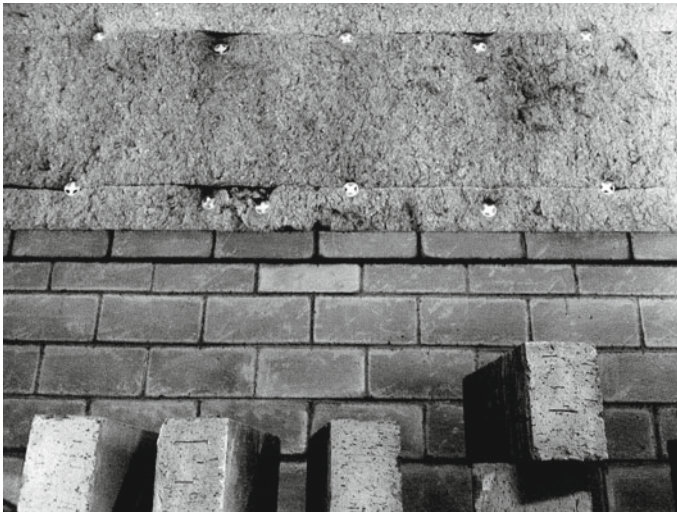
Fig. 2 Byo-construction system through compressed earth block and hemp insulation (photography). Source Author 2011
