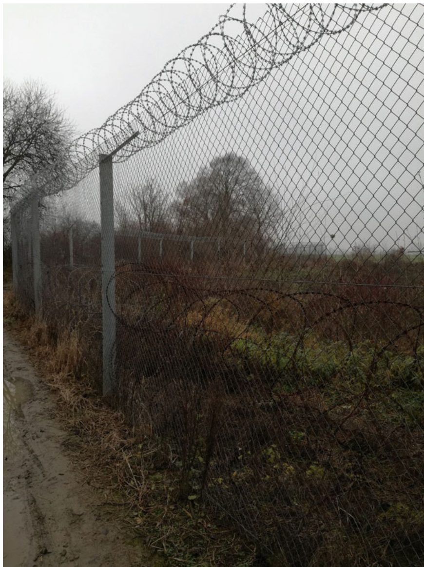
Fig. 6 Temporary security barrier for border surveillance purposes (2015). Source own photo
