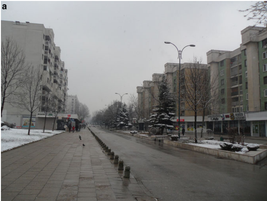
Fig. 13 Green pedestrian zone Bulevar Branilaca Dobrinje; Facades of Dobrinja’s buildings are dynamically designed, with large balconies, various kinds of opening, and more elaborate volumes. Source Elsa Turkusic Juric
