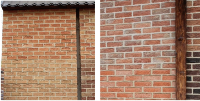
Fig. 3. Face ceramic brick based on medium-clay and clayey supports obtained by soft molding technology
