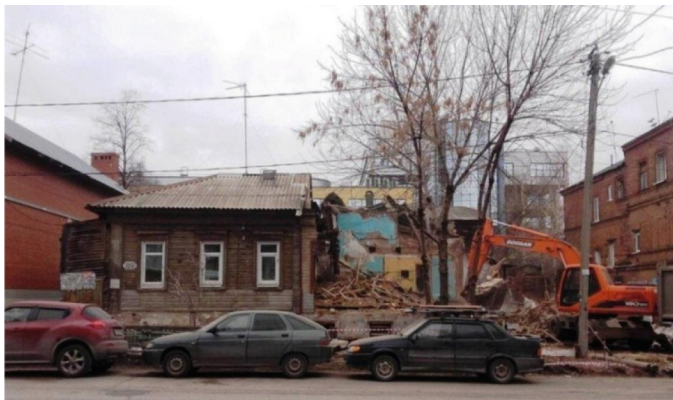
Fig. 1. Dismantling of buildings.
