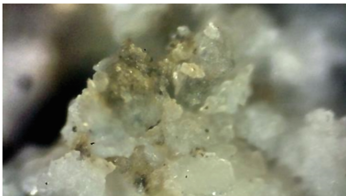
Fig. 4. Salt on the surface of the selected sample from the interior of the basement.
