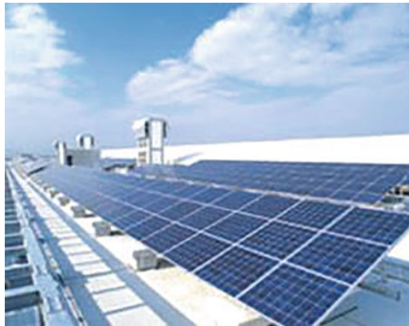
Fig. 2.12 Multi-crystal silicon solar cell
