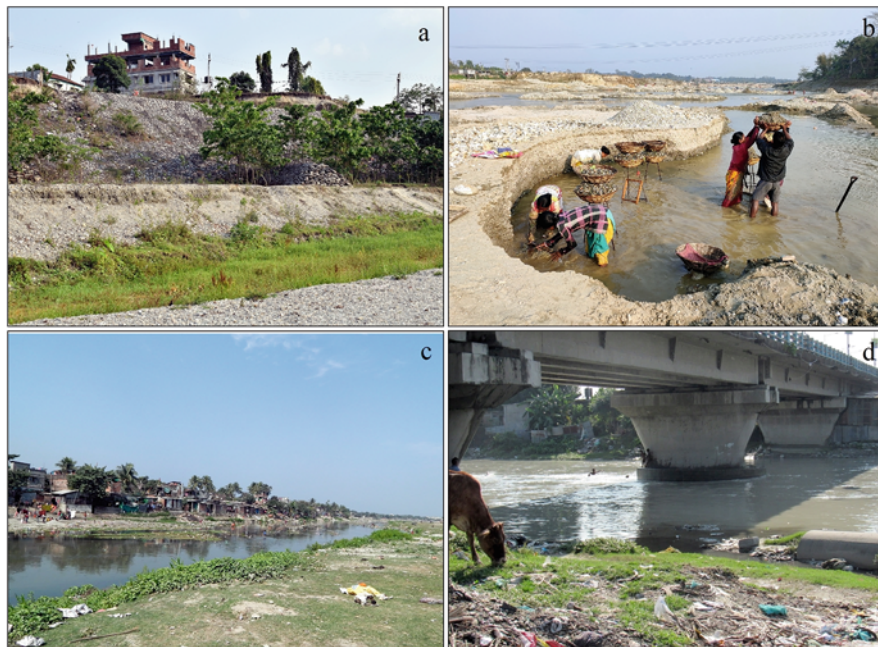
Fig. 6.6 Glimpses of ongoing anthropogenic interventions in the study area: (a) large embankments with groynes and bed stabilization structures along the banks of M, (b) intensive sediment extraction from the B river bed, (c) encroached banks of M, and (d) bridge pillars altering the flow of M. Pictures were taken by the author in December 2016 and April 2017. (Figure prepared by the author)
