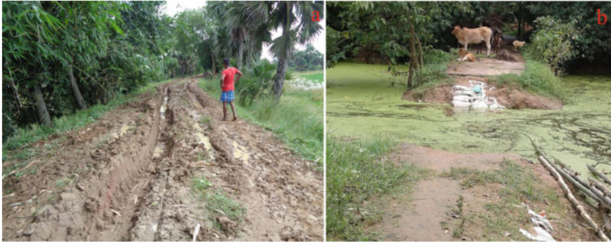
Fig. 10.6 Condition of the village road: (a) Typical katcha road during the monsoon and (b) breaching of the pucca road by flood. (Source: Field photographs, 2018)
