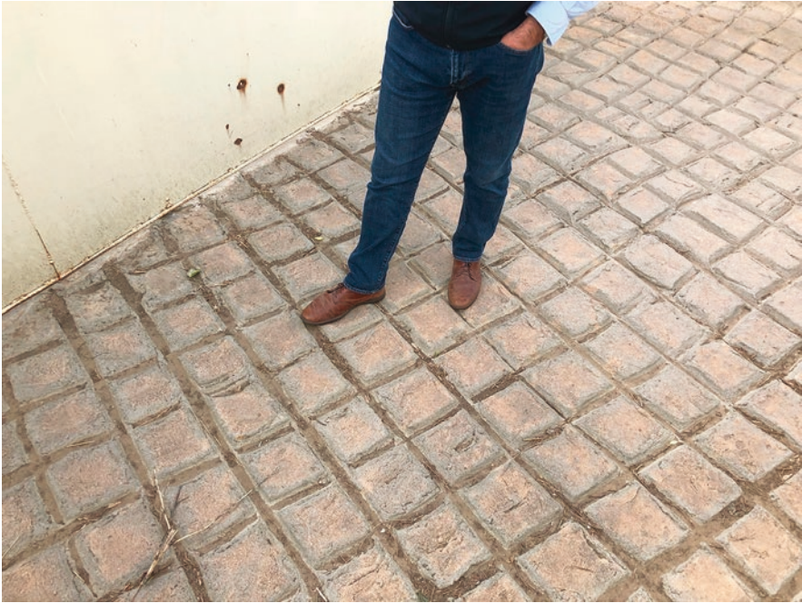
Fig. 8.3 Well-designed nonslip flooring for a cattle slaughter facility (Photo courtesy of Temple Grandin)
