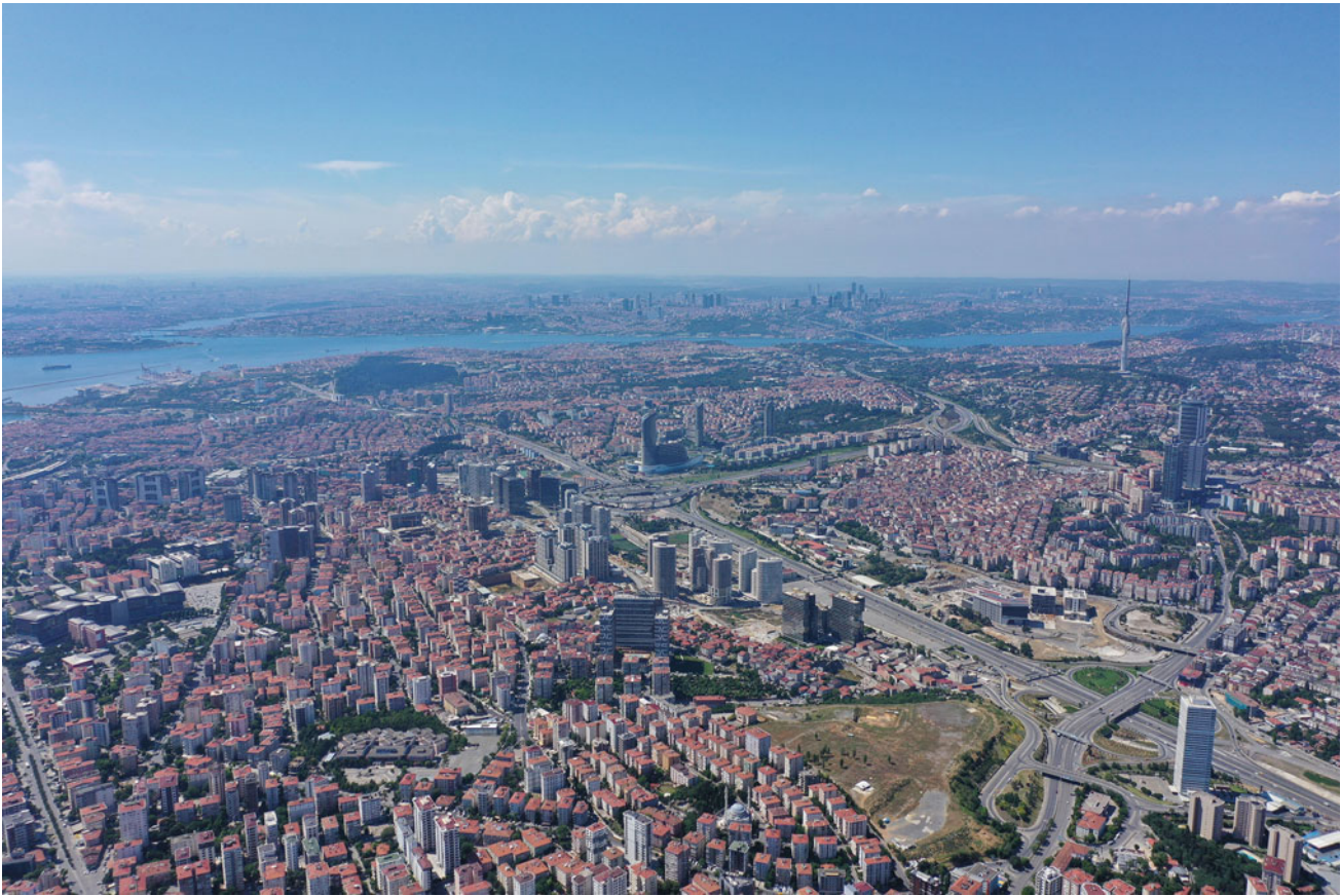
Fig. 7 Istanbul, large-scale regeneration project in Fikirtepe, Kadıköy District, in the scope of the earthquake plan will be applicate in the area of poor quality, slum houses, ( gece-kondu ), mid of the Photo, carried-out by mostly private construction companies. Photo, Fikirtepe.com
