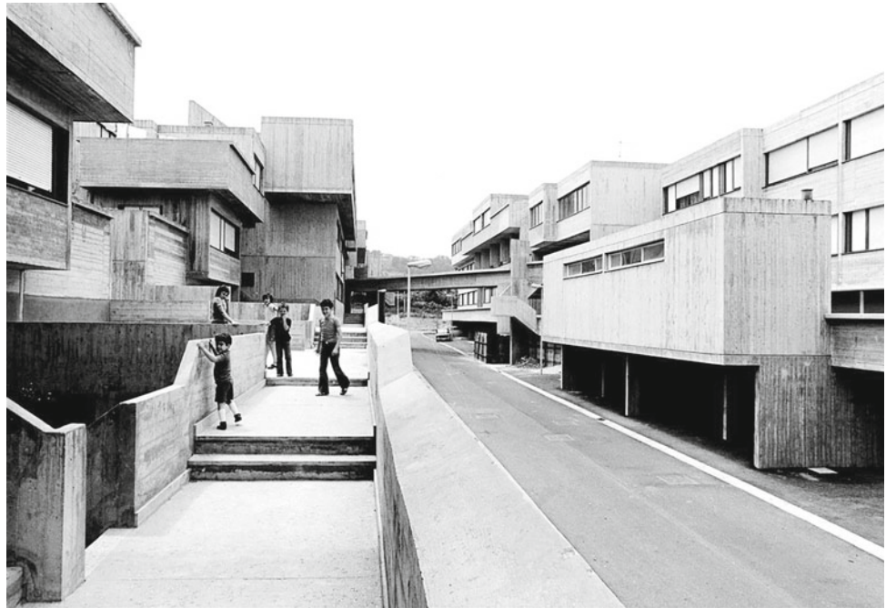
Fig. 4 The Villaggio Matteotti at Terni (Italy), designed by Giancarlo De Carlo (1975). Photo Giorgio Casali ( https://www.facebook.com/centrostudigiancarlodecarlo/ )
