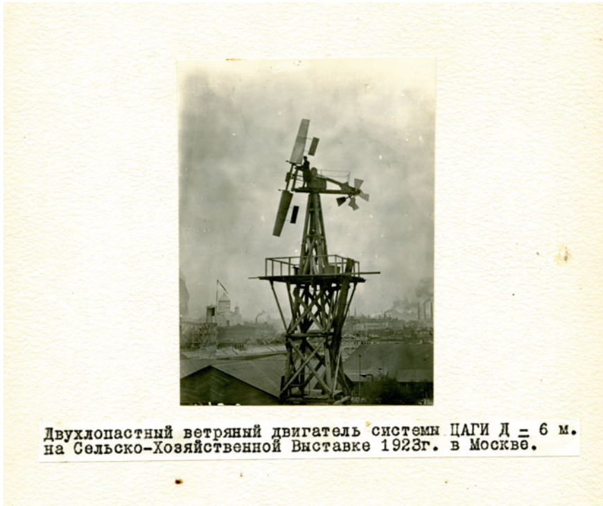
Fig. 11 TsAGI's experimental wind turbine at Zhukovskiy, near Moscow, 1923. Translation of text in Cyrillic script: Two-blade windmill-engine system (= wind turbine). TsAGI D = 6 m. At the 1923 agricultural fair in Moscow. Photo Jos Beurskens Collection
