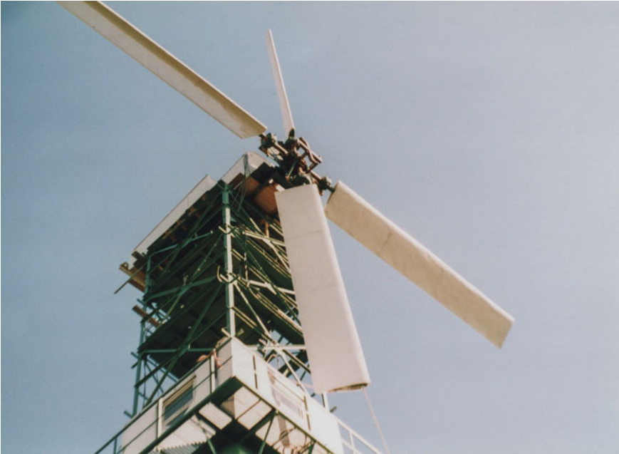
Fig. 26 Wind turbine built by Martin Unger in 1973, Forstwolfersdorf, (GDR). In the German Wind Energy Museum. [Foto used with permission of Martin Unger]
