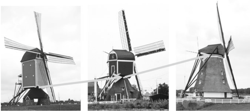
Fig. 6 The development of the classic “Dutch windmill”. Photos Jos Beurskens
