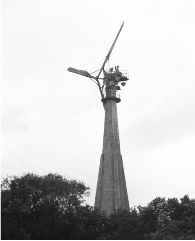
Fig. 13 A decommissioned Smidth aeromotor in Denmark. Rotor diameter 24 m, rated power approx. 70 kW. The picture dates from 1972. Photographer Paul Smulders
