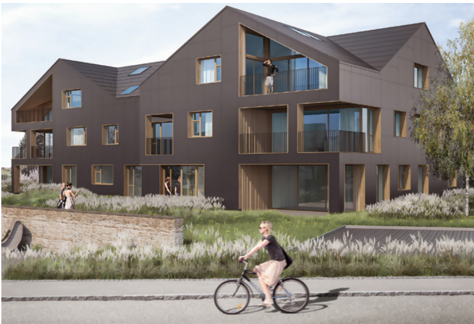
Fig. 8. Self-contained multi-family construction project (ZEB) https://www.umweltarena.ch/
