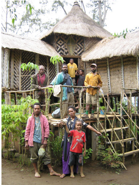
Fig. 7.5 A ‘castle’ in Papua New Guinea, fabricated from palm trees and some tropical timber, and earthquake-proof
