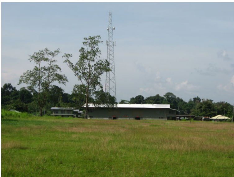
Fig. 4.11 Typical 'station': a hub of rural live in Papua New Guinea centered around a phone tower and a landing strip
